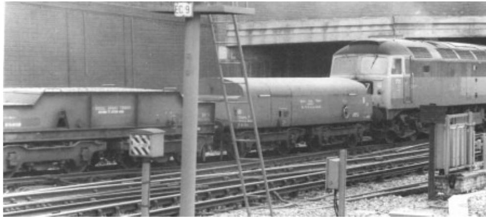
When diesel locomotive haulage of unfitted goods trains was first introduced, it was considered that the locomotives would have insufficient brake power to control their trains, so some special "diesel brake tenders" were introduced. These were heavy wagons (35½ - 37½ tons) fitted with automatic vacuum brakes. On some BR Regions they were usually pushed by the loco, but on the Southern Region it was normal practice to pull them.
