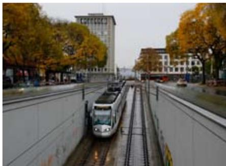
Tram-trains access Kassel's tramway via this specially-designed 'dive-under', which passes beneath the forecourt and concourse of the main station...
