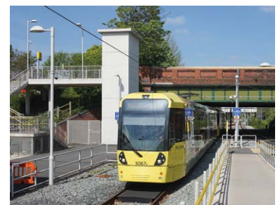
▲ Completed in 2013, the South Manchester Line redeployed the Midland Railway route where tracks had been removed in 1970. East Didsbury terminus adjoins a park-and-ride.
