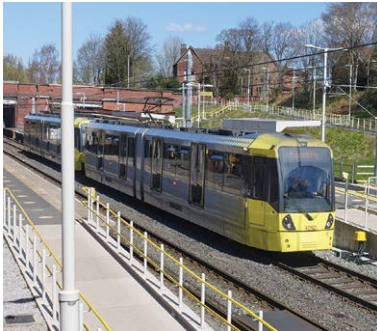
◀ LEFT: Recently rebuilt to add a turnback facility for future use as a terminus, Crumpsall on the Bury line retains many original railway features, yet illustrates the works needed to improve access for light railway use.
