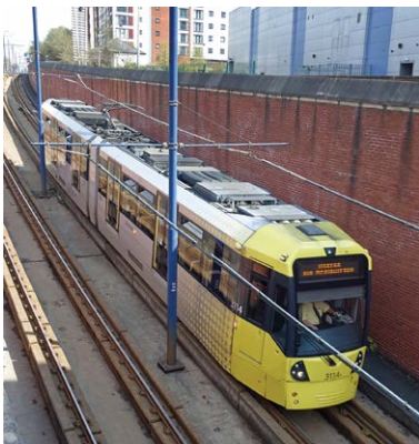
▲ ABOVE: Much of the first extension, the Eccles line, shares road space. This underpass avoids conflict at an intersection between Ladywell and Eccles terminus.
