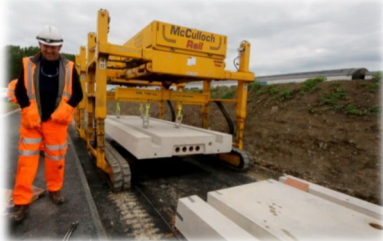
*Precast Advanced Track Installation less than £10M per Km
