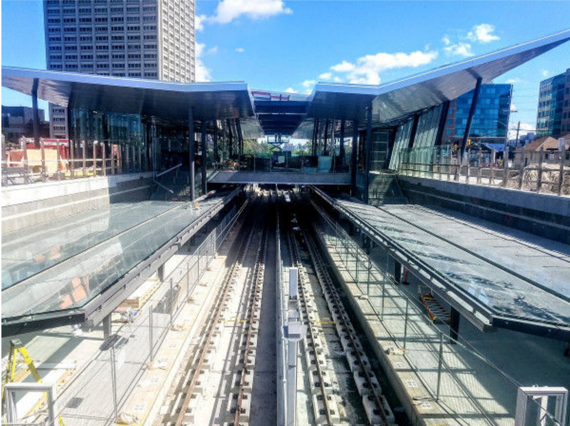
Tunney's Pasture LRT Station looking west October 4, 2018 (Image Credit: Fraser Pollock)
