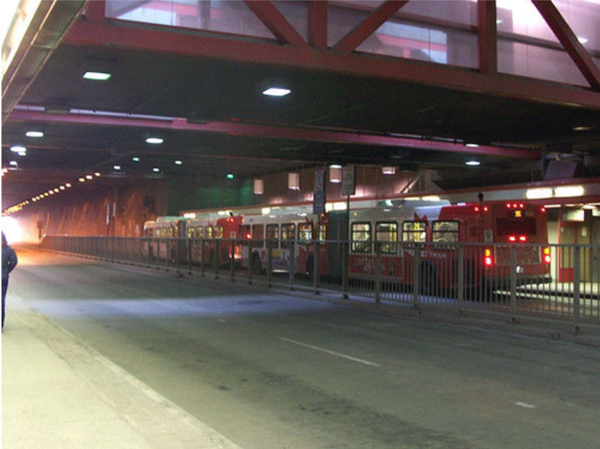
St. Laurent Transitway Station before conversion to LRT, looking east. (Image Credit: O.C. Transpo)
