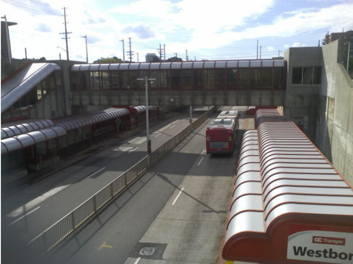
Plastic panels on Westboro Station roof (Photo Credit: Fraser Pollock)
