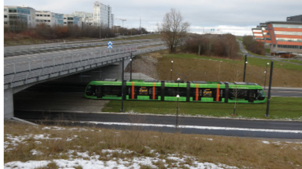
▲ ABOVE: Tramway installation required a new bridge for the E22 motorway, moved into place on 9 April 2018. The E22 is used by 40 000 cars on a normal day.
