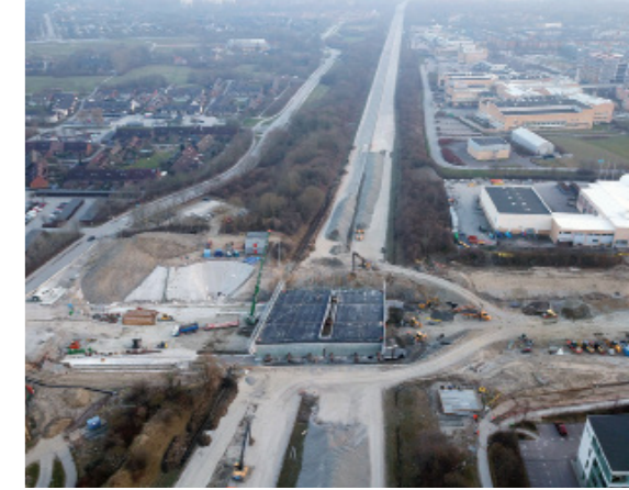
▲ ABOVE: Tramway installation required a new bridge for the E22 motorway, moved into place on 9 April 2018. The E22 is used by 40 000 cars on a normal day.
