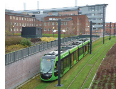
▲ ABOVE: The underpass at Tornavägen was built for the busway in 2002, featuring a nice brick wall design.
