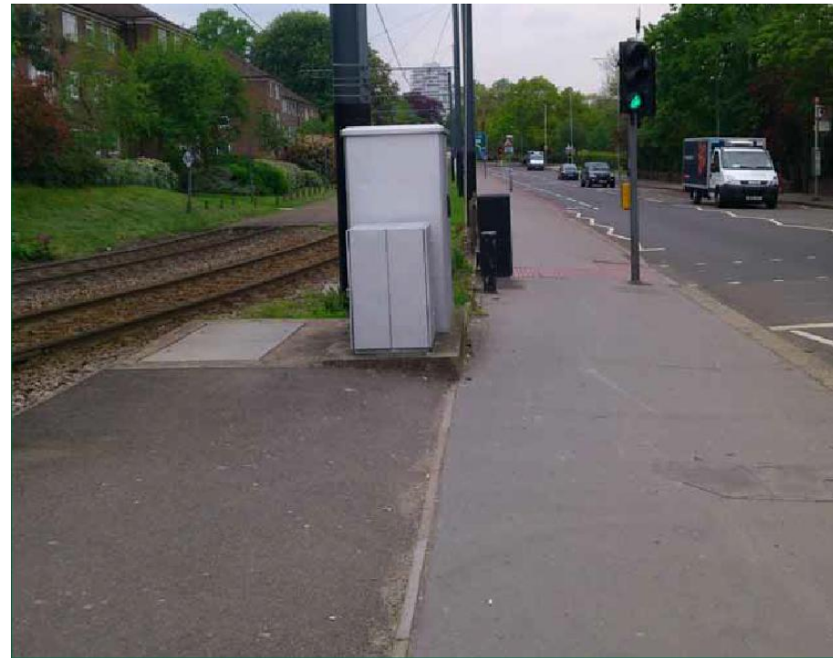
Figure 5: The obstruction to the pedestrian's view of approaching eastbound trams at Sandilands tram stop
