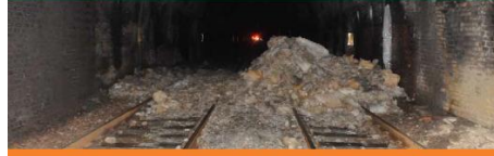
Derailed in Summit tunnel, near Todmorden, West Yorkshire 28 December 2010
