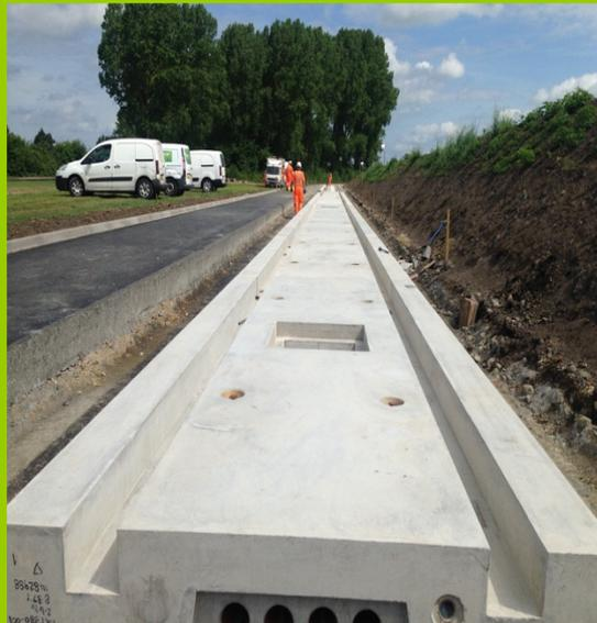
If needing to replace utilities, slabs can be **easily removed** and repairs done.
