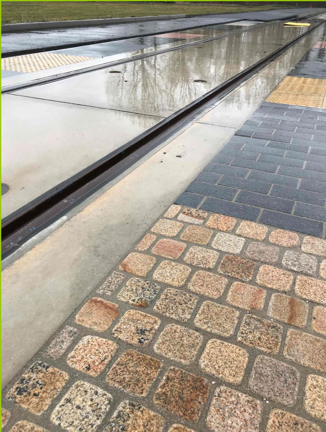
The high strength PCAT precast slabs reduces construction depth by **over 50%**
