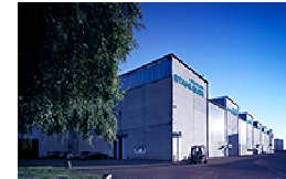
Stadler Stahlguss 120 employees
