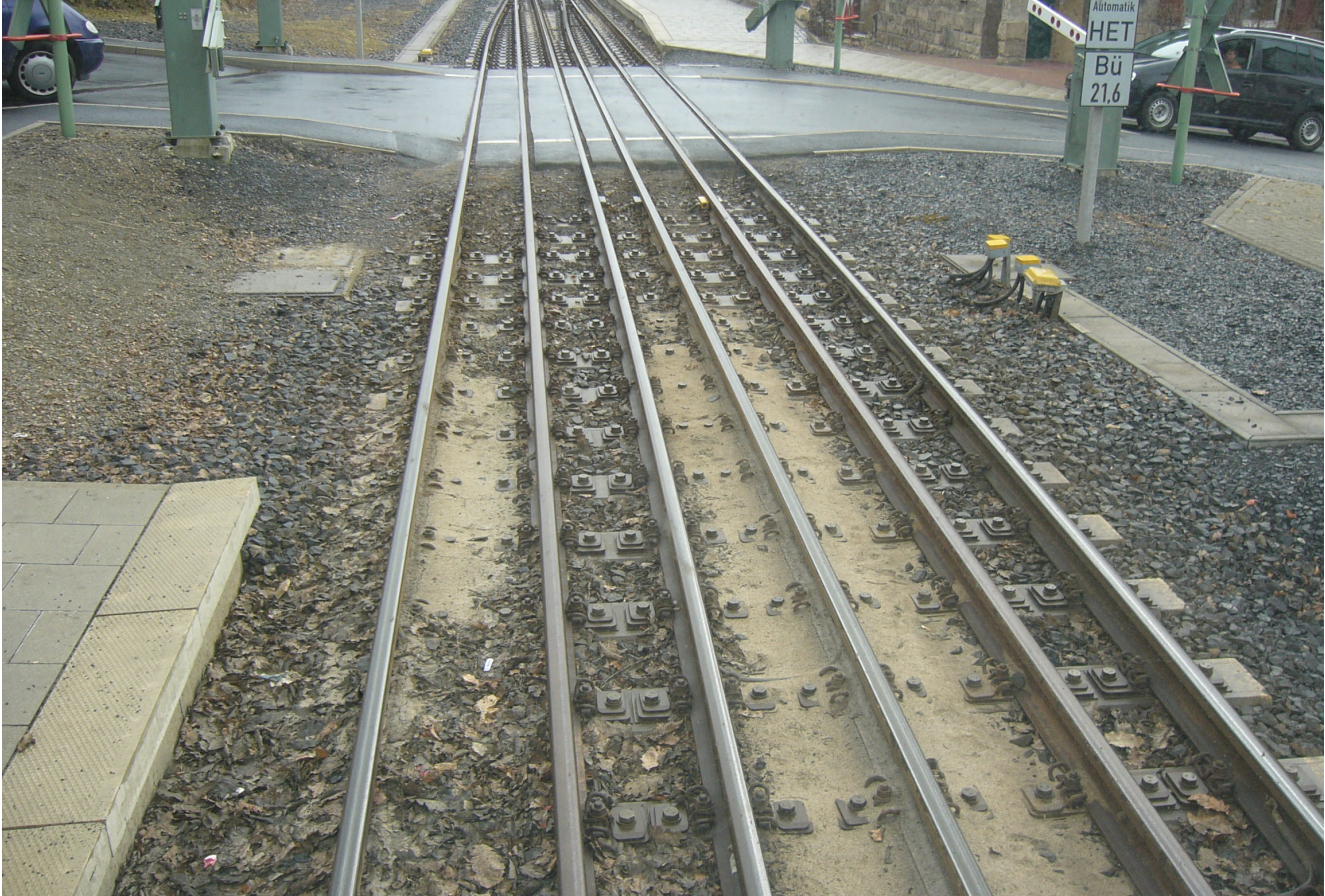
A simple but ingenious solution to mixed gauge bodies on the Kassel TramTrain system
